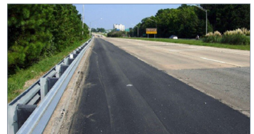
Example of stiffened guardrail placed along curb. Source: Kimley-Horn.
