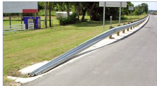
Anchorage located at trailing (downstream) end of traffic barrier. Source: Kimley-Horn
