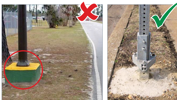
Improper and correct usage of a breakaway device.
