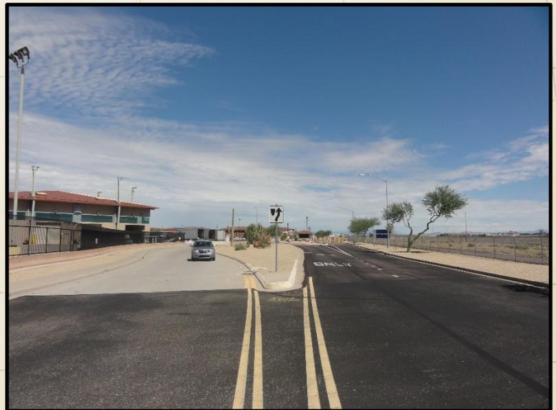
Where islands are smaller, painted islands can be used to delineate the travel path. Similar pavement markings are used versus those with a raised island, however hatching can be used to discourage travel over the island.
