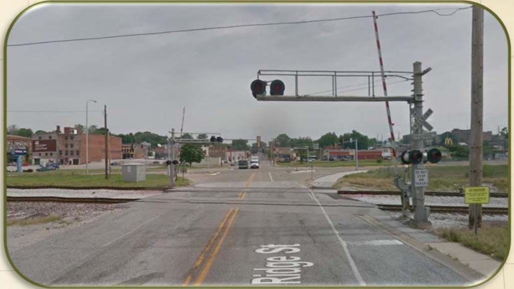
The actual intersection of a roadway and railroad should be as level as practical. Vertical curves should be of sufficient length to provide an adequate view of the crossing.
