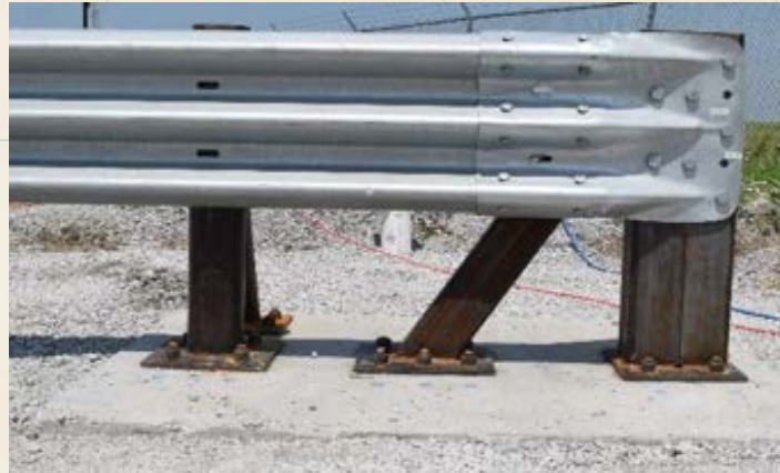
Rear View of End Anchor
