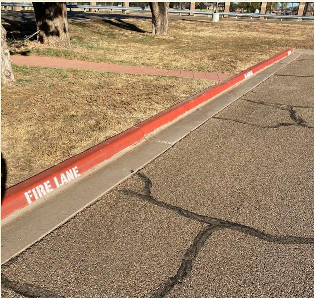
requires that an 18 by 24-inch sign stating NO STOPPING FIRE LANE be marked at the entrance to the property facing incoming traffic. Additionally, the code requires that fire lanes be marked by one of three options:
