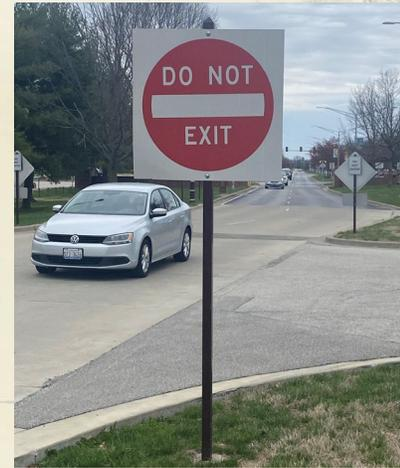
This photo illustrates an alteration of the standard DO NOT ENTER (R5-1) sign panel used at a site access, violating the MUTCD. At a glance, this sign is easily misinterpreted.
