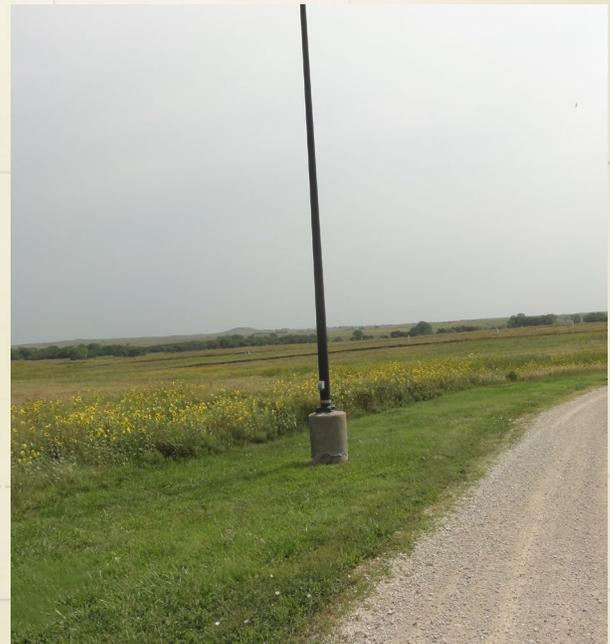
This photo illustrates a light pole foundation extending approximately 4 feet above ground in the clear zone
