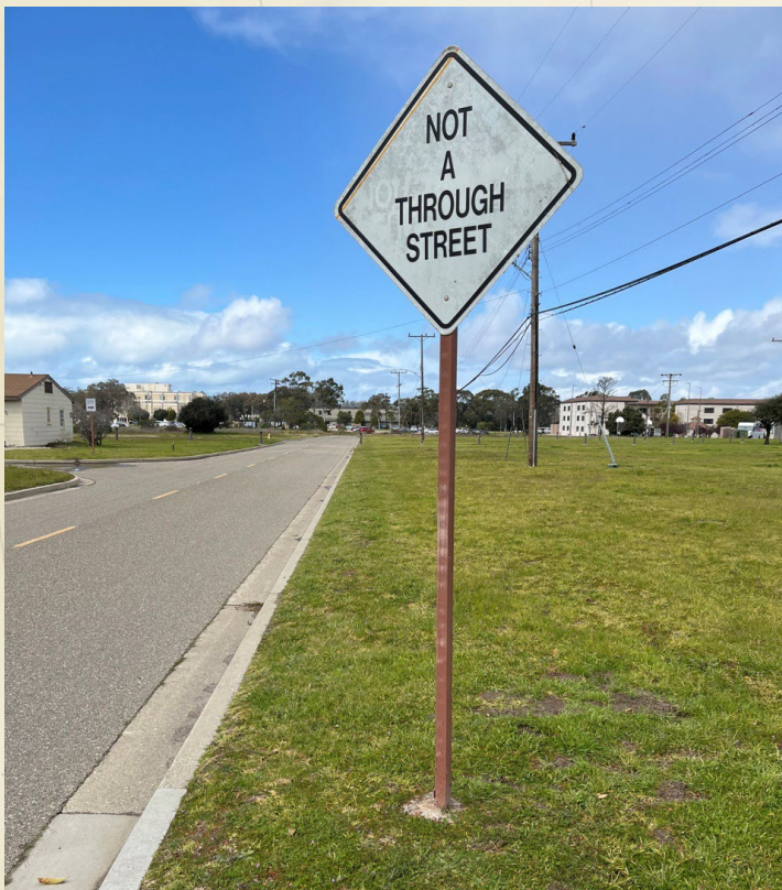
Example of Faded Sign. Also, note that the background was used for another sign previously.
