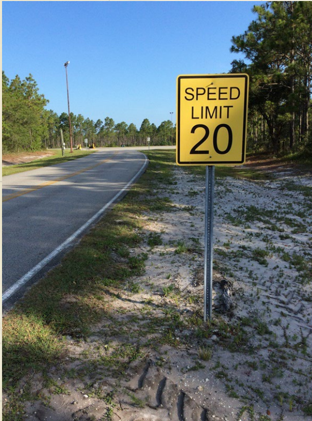
Example of Incorrect Color for Speed Limit Sign
