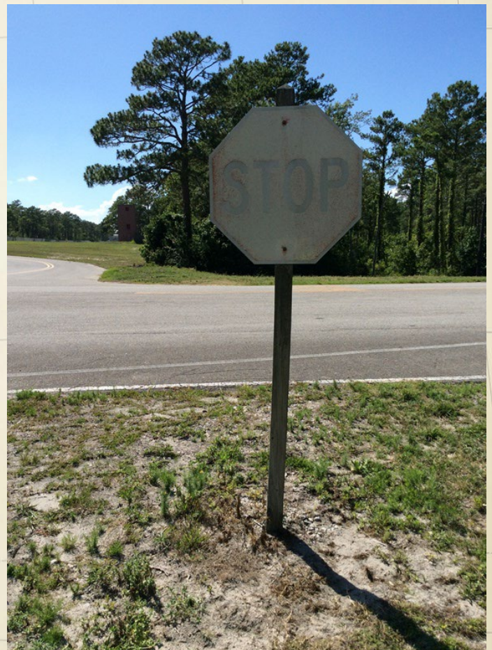
Example of Faded STOP sign
