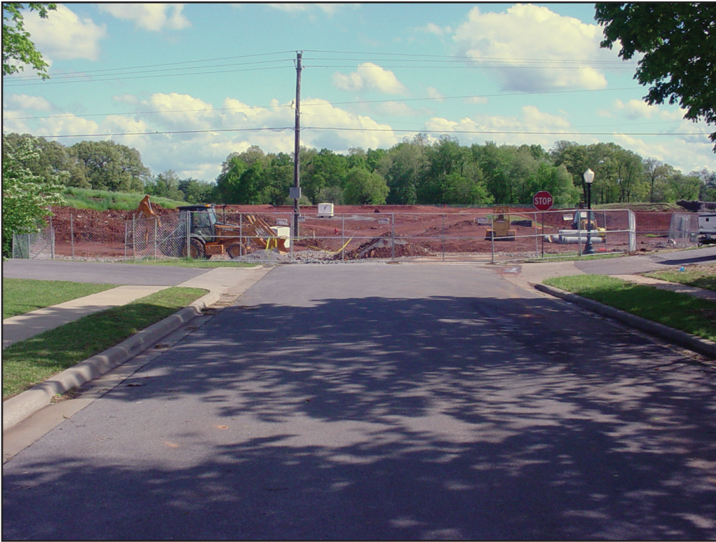
Work zone involving a closed roadway with no signing to indicate the closure of the roadway
