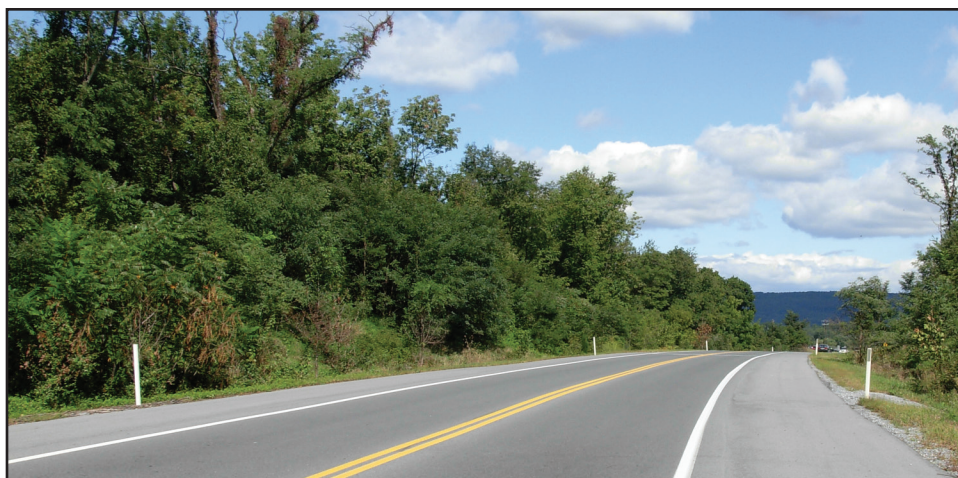
Proper use of delineators
