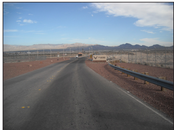
Non-Retroreflective RPMs
