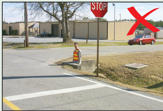
Endwalls too close to roadway edge for cross-drainage structures
