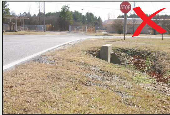
Protruding endwalls for cross-drainage structure
