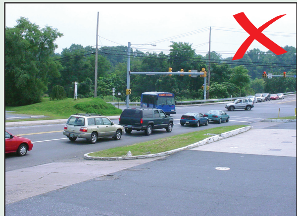
Driveways too close to a signalized intersection become blocked by stopped vehicles.
