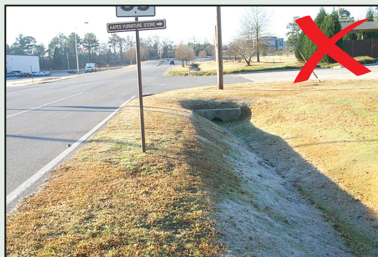
Parallel-drainage ditches within the clear zone Note: Parallel ditches are not an obstacle if properly designed.
