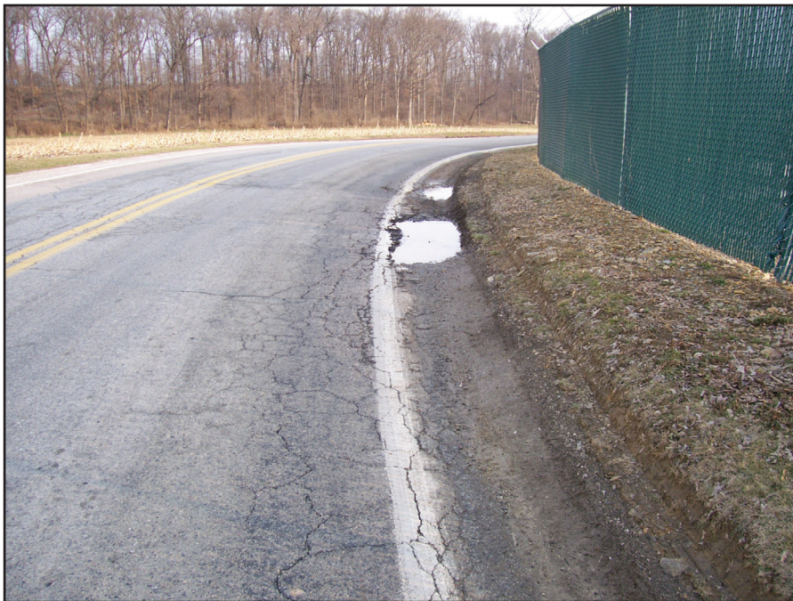
Poorly maintained shoulder
