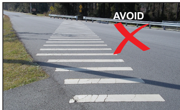
Exhibit 8.15: Skewed Crosswalk Configurations
