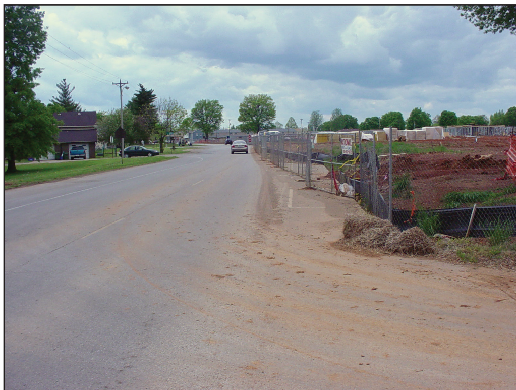
Work zone lacking proper tapers, signing, and temporary pavement markings
