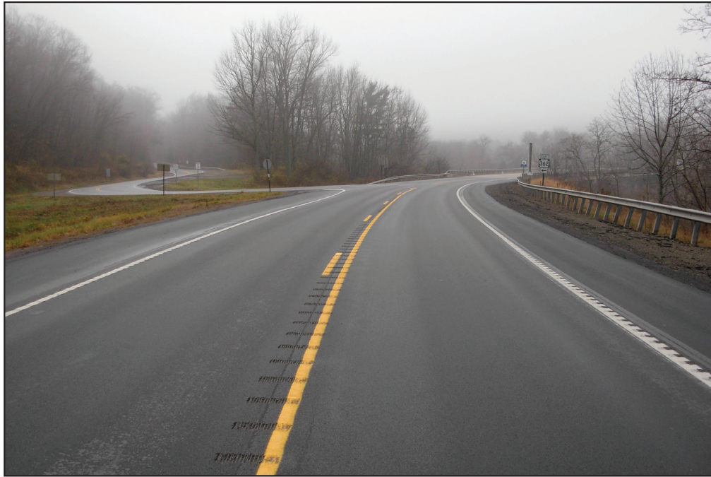
Shoulder and center line rumble stripes
